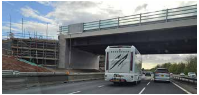
The new bridge spans the M4
