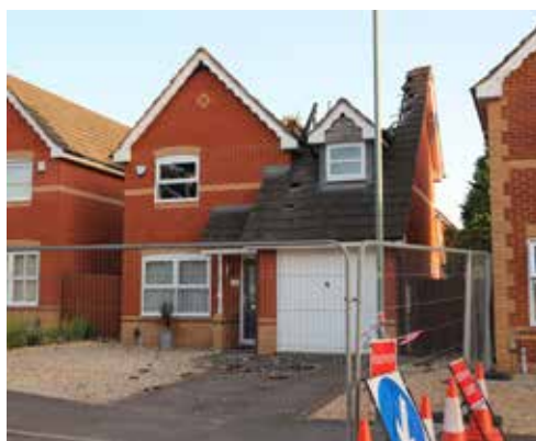
The home in Wadham Grove was wrecked after being hit by lightning.
